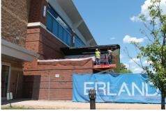
Erland returned to Electrochem's headquarters in Raynham, after an explosion in one of their testing labs, to immediately investigate the safety of the structure. Partnering with ahp Architects on this design/build effort, a new structurally retrofitted material testing room was constructed. The 12-inch thick walls are structurally reinforced vertically and horizontally to withstand an explosive force.
